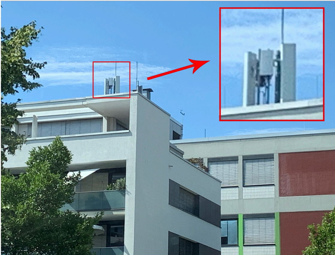
5G 3.5 GHz Cell Site of Deutsche Telekom in Darmstadt, Germany
